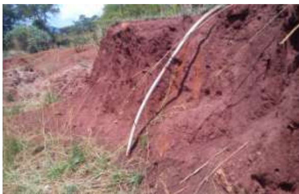
Figure 12: Land degradation threatening water pipe in Guruve
